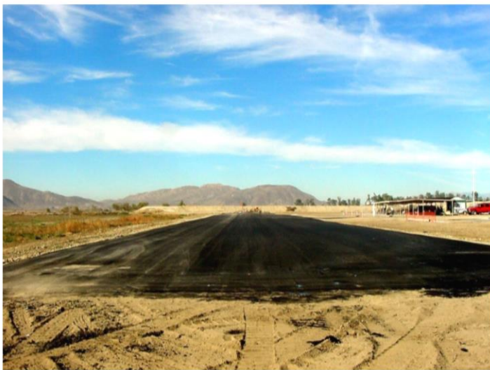
Asphalt Paving being put down at the relocated runway on November 21, 2002.
