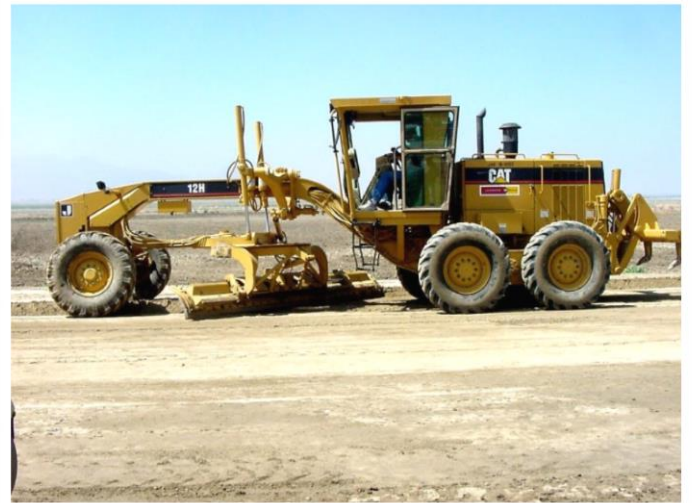
Mark Jarrell grading our relocated runway on June 2, 2002.
