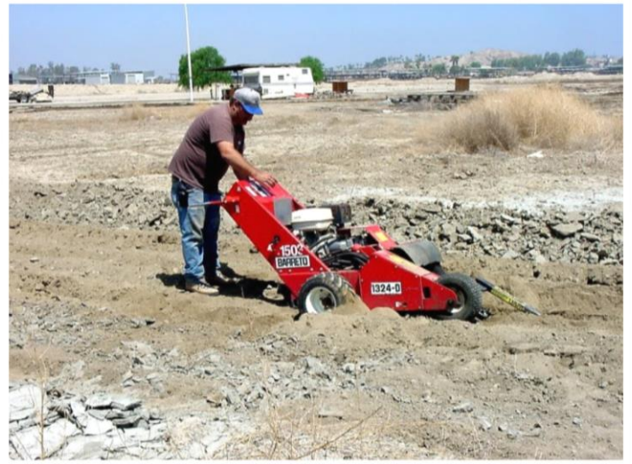
Dave Hollingworth operating a Ditch Witch, digging a trench for running electric and water lines to the relocated runway in June 2002.
