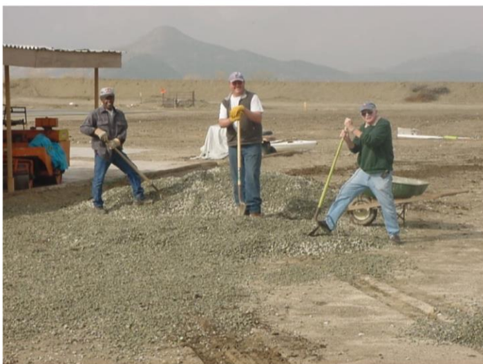
Roy Truitt, Jeff Vanderpol, and Mel Santmyers spreading gravel in the parking area of the relocated runway on February 14, 2003.
